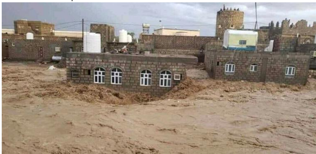
Photo 1: Flood impact on houses.
