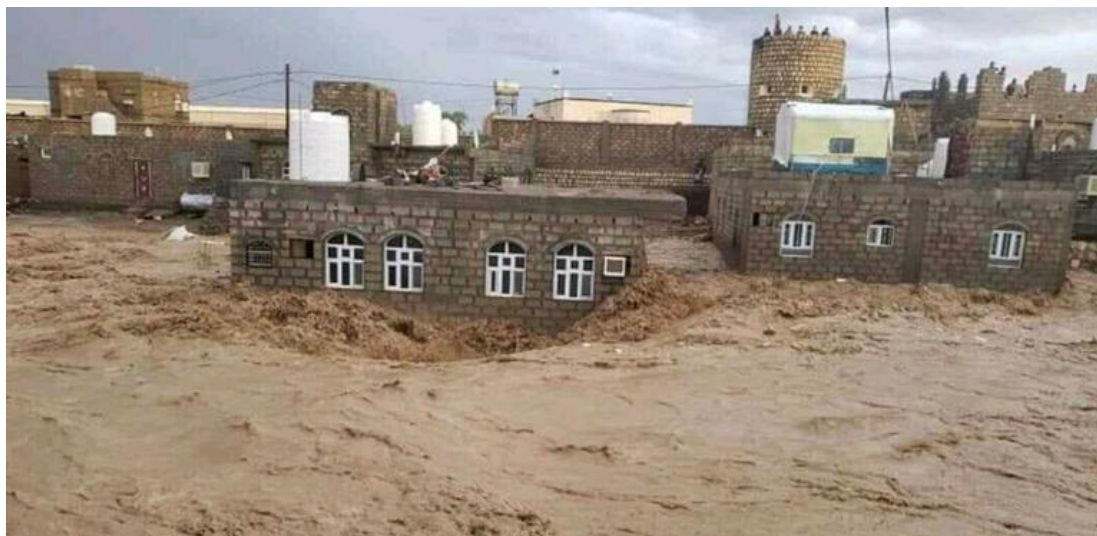
Figure 9: Flood impact on houses
