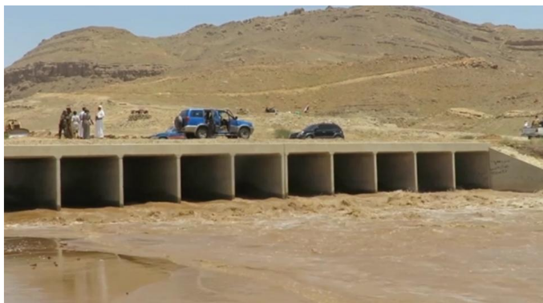
Figure 10: Flood management structures.
