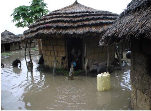
Fig 3: A grass thatched house destroyed by floods
