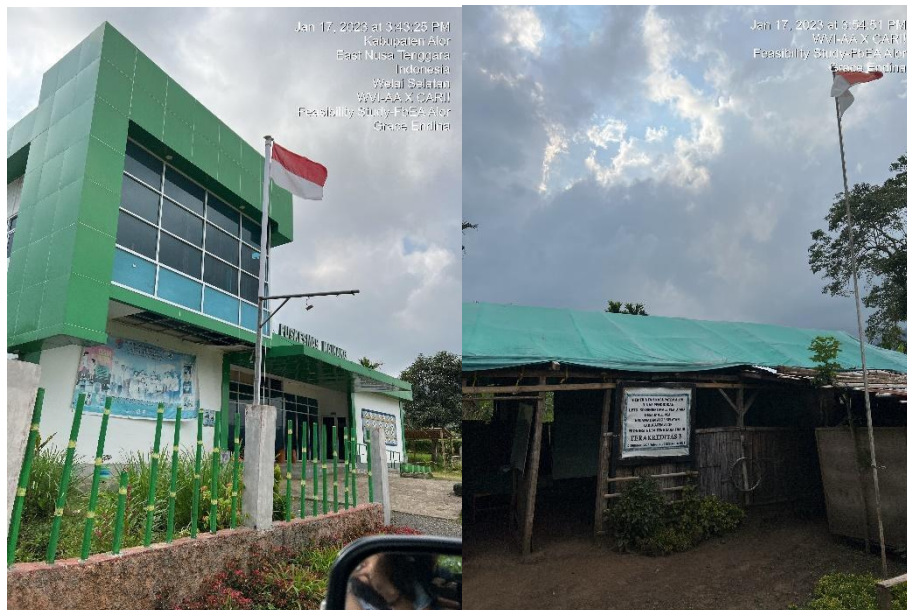
Figure 46 Health facility remained intact (left) and temporary elementary school (right) due to the Seroja 2021
