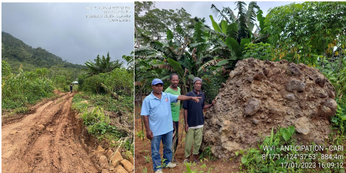
Figure 45 Neighborhoods in Malaiepa village were wiped out during the Seroja 2021
