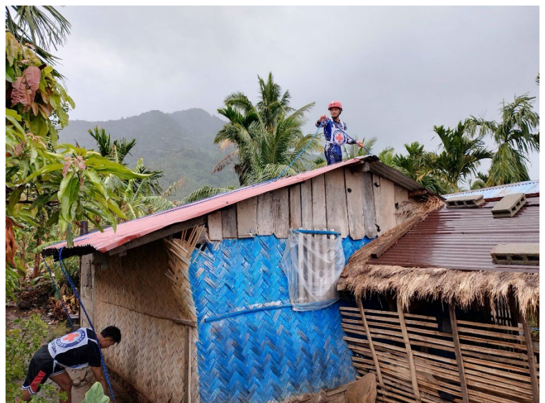
PRC personnel installing Shelter Strengthening Kits in Aurora Province (Photo: PRC)
