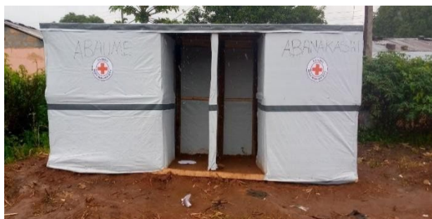
Temporary latrine constructed in Ndola Mapalo camp ©ZRCS
