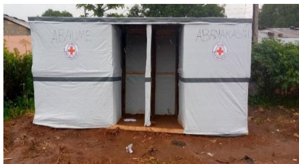
Temporary latrines constructed in Ndola @ZRCS
