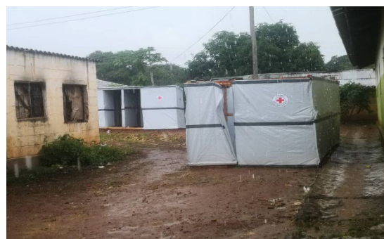
Temporary bathrooms constructed in Maplo camp @ZRCS
