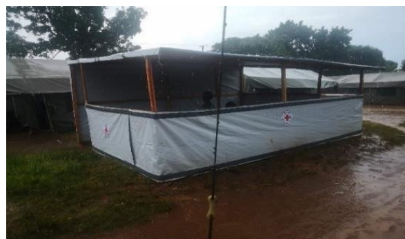
Temporary Kitchen shelter constructed in Ndola ©ZRCS
